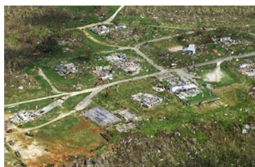
Damage from Supertyphoon Pongsona on the island of Rota, 20 December 2002. Image courtesy FEMA Photo Library, Andrea Booher.
